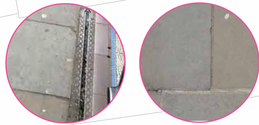
Yorkstone flag stones and traditional iron drainage channels
