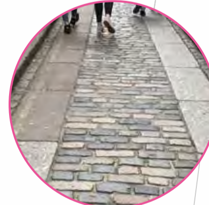
Cart wheel stones laid into cobbled carriageway
